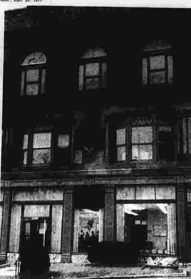
This building, built in the 1800s, has a rare cast iron front and will probably be included in a survey being prepared for a grant proposal by the Vernon Historical Society. The building is on Elm Street and has been bought by the Union Congregational Church which is next door. (Herald photo by Richard J. Dodds)
